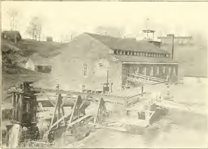
FIG. 2.—LEAKSVILLE COTTON MILL, ON DAN RIVER, SPRAY, N. C., BUILT IN 1839.
